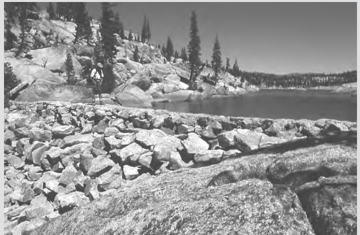
Though the Forest Service claims that dams in the Emigrant Wilderness serve the recreational, scenic, scientific, educational and historical purposes of Wilderness, a federal court correctly found that rebuilding or operating the dams is unlawful because would be contrary to the purpose of the Wilderness Act.
